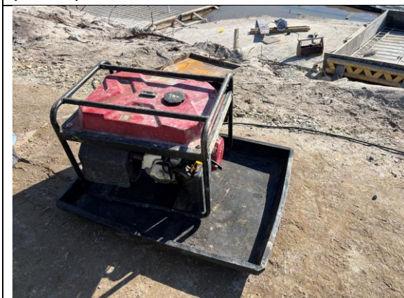
PHOTO 23: Generator on site with drip tray
