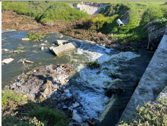
PHOTO 33: Future work area where the fishway will be constructed
