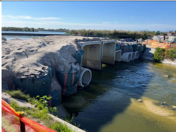
PHOTO 31: Water flow is ensured past the work area
