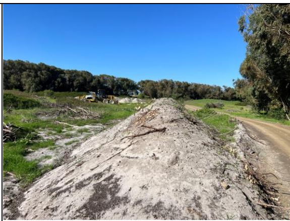
PHOTO 20: Topsoil stockpiled for later use
