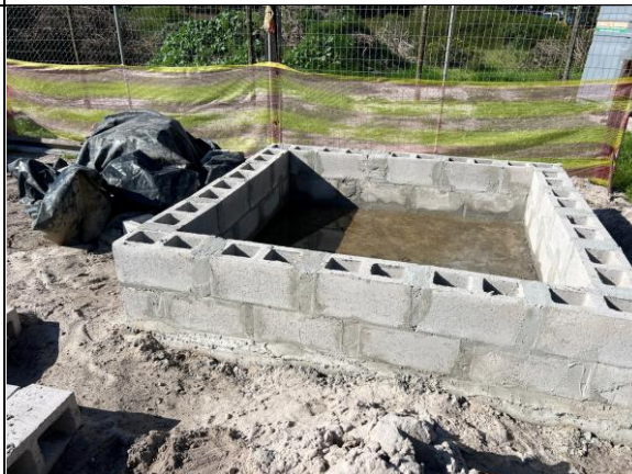
PHOTO 22: Additional bunded storage area constructed
