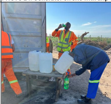
PHOTO 26: Drinking/wash water on site
