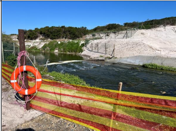
PHOTO 32: Downstream of the work site
