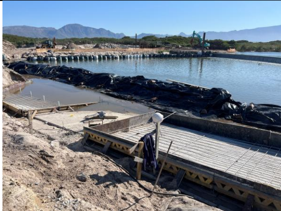
PHOTO 29: Concrete works in the foreground and cofferdam in place behind; contained water requires management in accordance with the approved MS
