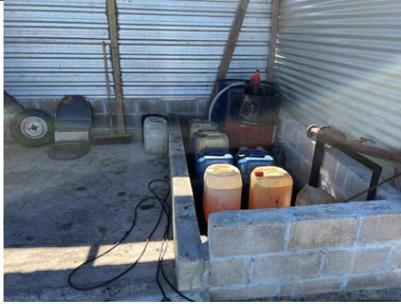
PHOTO 1: Bunded and covered area for parking of diesel bowser and liquid hazmat drums
