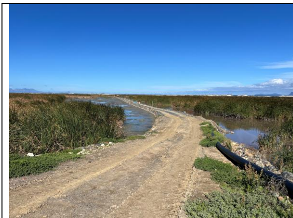
PHOTO 7: Bund wall over S3 Pond
