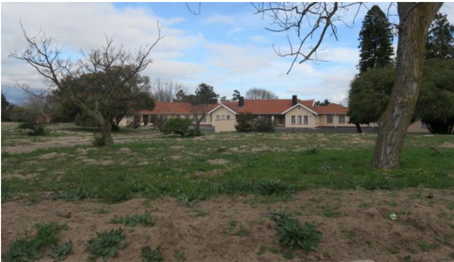
Figure 112: The rear of CMHP
