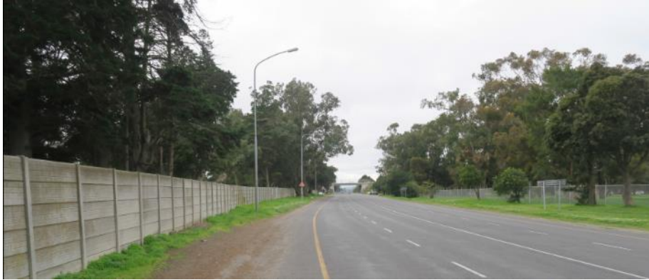
Figure 15: Tree line along Old Paarl Road in proximity to the intersection with De La Haye Avenue, Stikland north left, behind the vibacrete wall and Stikland South right
