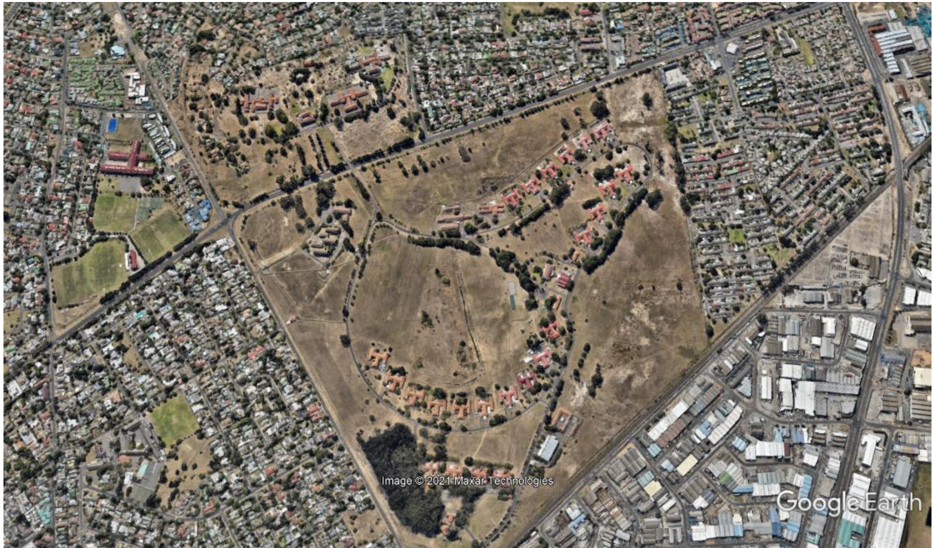
Figure 67: Stikland Psychiatric Hospital site (Google image 2021), virtually unchanged since it was constructed
