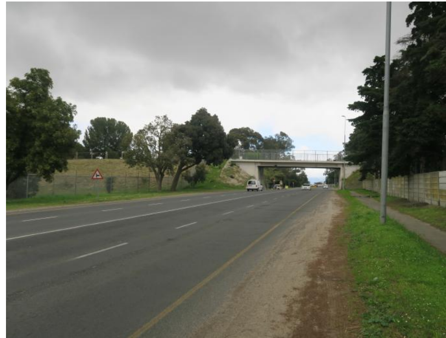
Figure 118: The R301 as it passes through Stikland Hospital, Stikland South to the left; Stikland North to the right, the disused bridge connecting the two.
