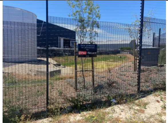
PHOTO 10: Southern attenuation facility, banks are stabilised
