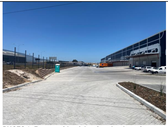
PHOTO 8: Eastern side of the site – landscaping evident
