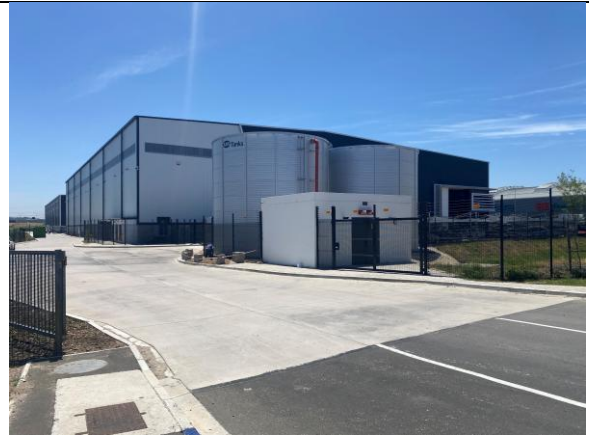
PHOTO 2: Site entrance off Cilmor Street
