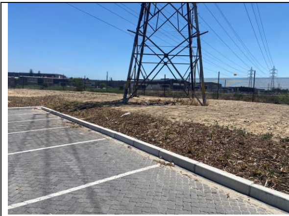
PHOTO 7: Landscape planting along the edges of the northern roadway. Note the area behind has been seeded, but vegetation cover still needs to establish.
