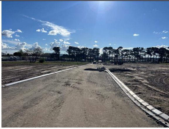
PHOTO 13: Site looking north - clean and tidy
