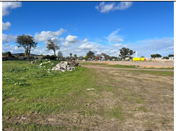
PHOTO 10: Legacy rubble stockpiles from previous contractor awaiting disposal
