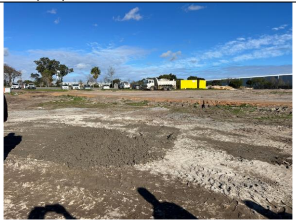
PHOTO 18: Designated kerb mix area which is lined with DPC plastic
