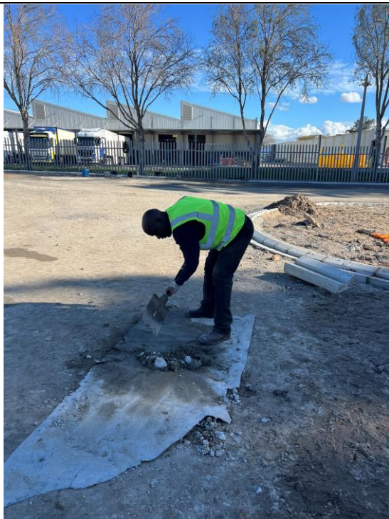
PHOTO 17: Careful cement product handling
