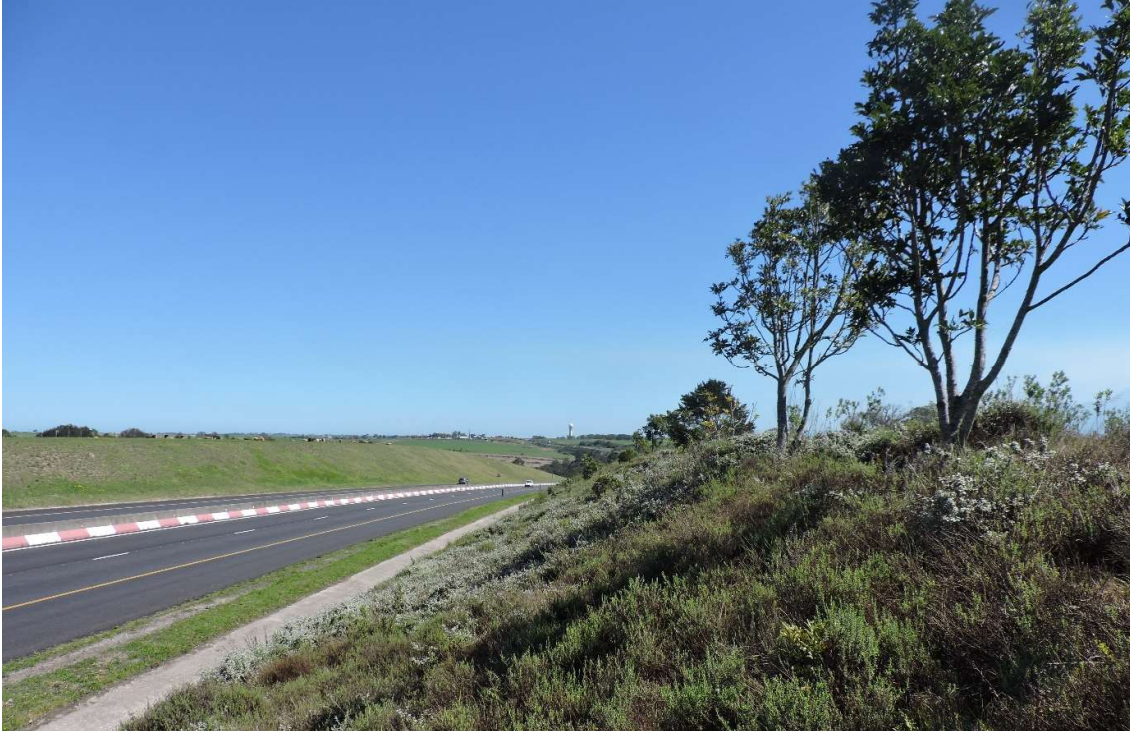
Figure A7: View of the eastern embankment which will be partially removed in case Alternative 1 is selected. The trees are Harpephyllum caffrum which were planted as part of the previous revegetation activity.
