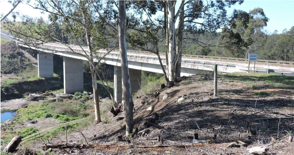
Figure A1: View of the northern (upstream) side of the bridge. The Eucalyptus trees (exotic species) will have to be removed in case Alternative 1 is selected.
