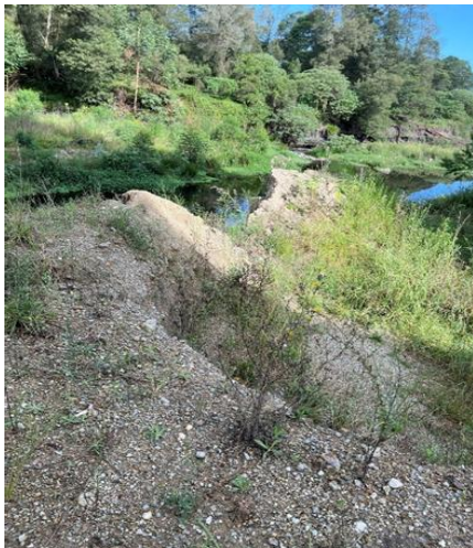
Photograph 20: Showing earth berm along the channel
