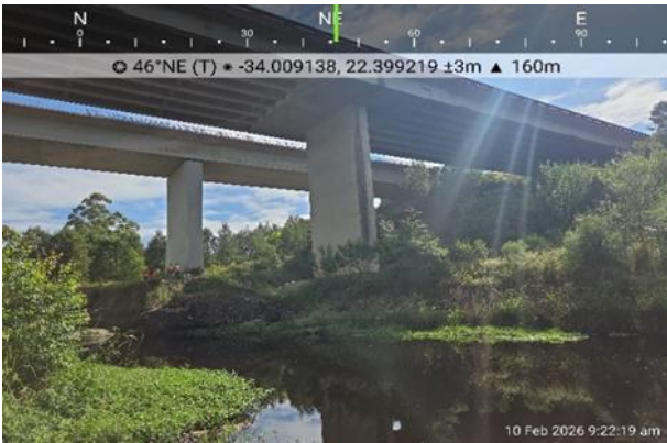
Photograph 1: Showing two completed eastern spans and pier above Gwaing River
