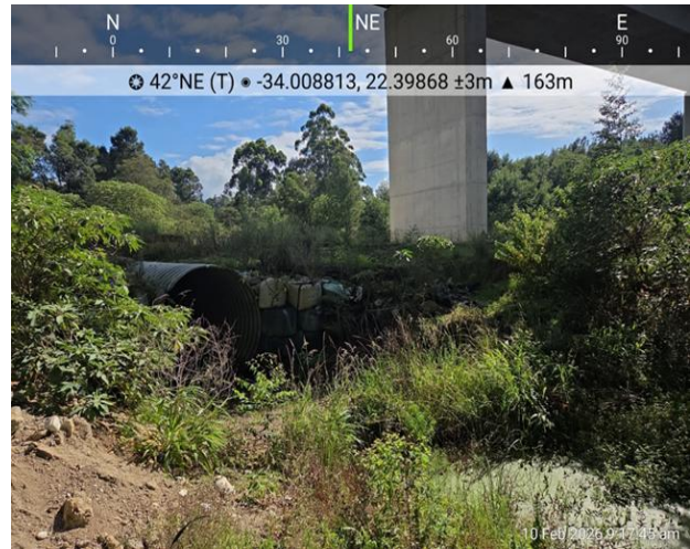
Photograph 21: Showing corrugated steel culvert temporarily conveying the river flows
