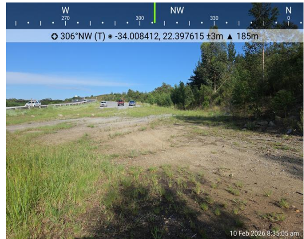
Photograph 15: Showing unfinished portion of the western approach
