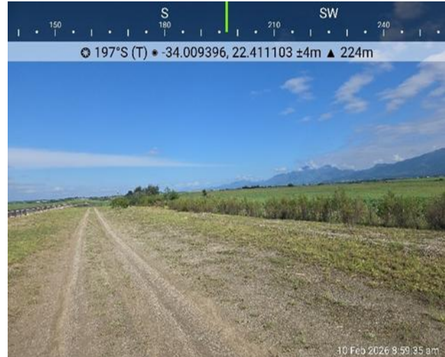
Photograph 7: eastern side of the approached constructed to subgrade level
