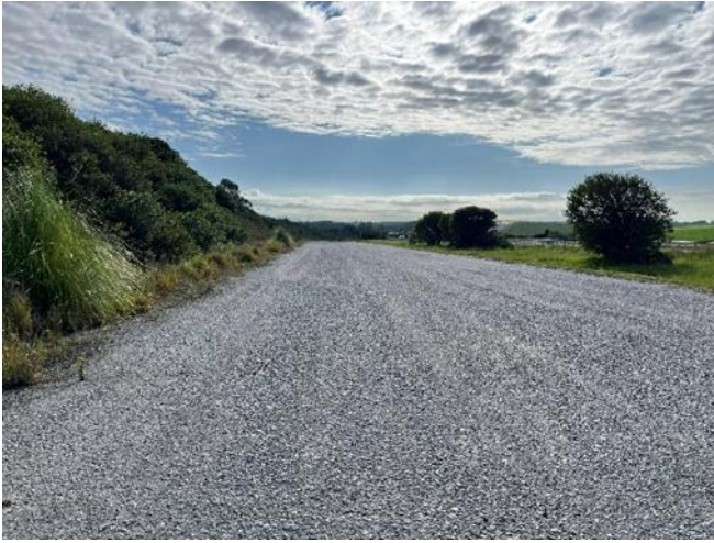
Photograph 9: Base layer partially completed on the western side of the bridge
