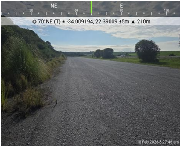
Photograph 14: Showing western approach road alignment completed to base level
