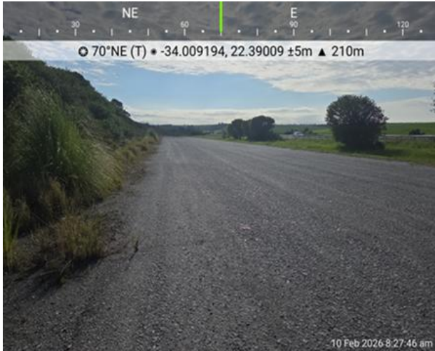
Photograph 6: Showing western side of the approach constructed to base level
