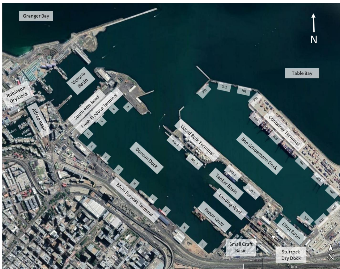
Figure 3.4. Aerial view of the Port of Cape Town, showing the positions of the Victoria and Alfred (V&A) Basins, the Duncan Dock and Ben Schoeman Dock, as well as Table Bay and Granger Bay (Google Earth 2023).
