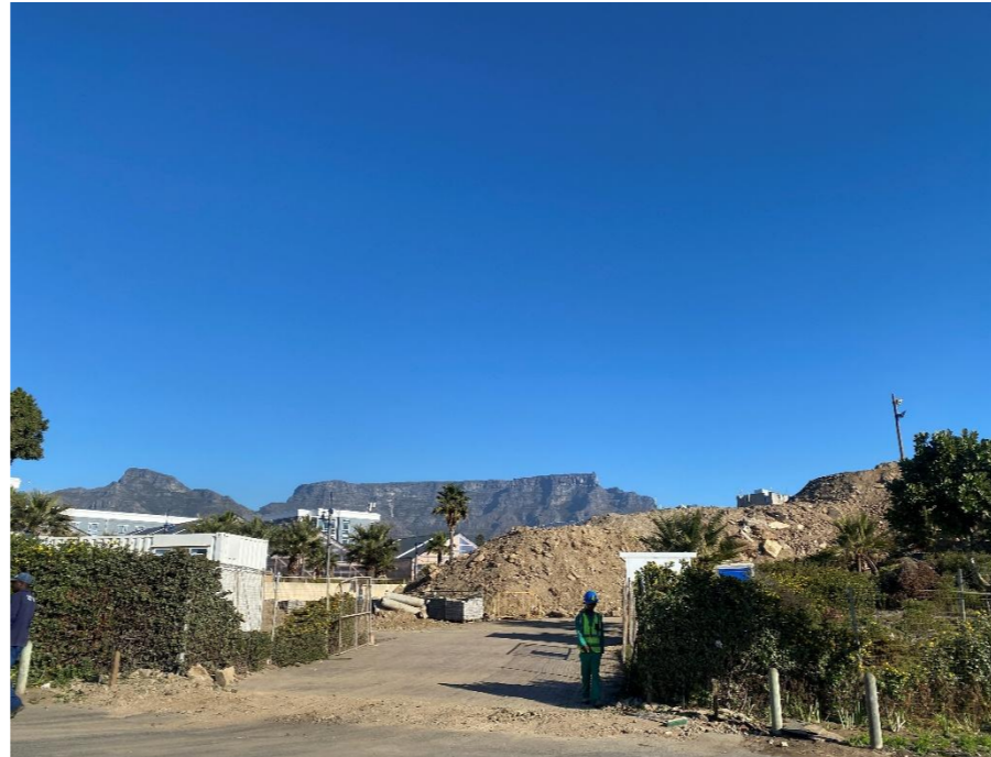
Photograph 3-8: View of the Construction spoil area on site (location of the previous The Lookout Venue)
