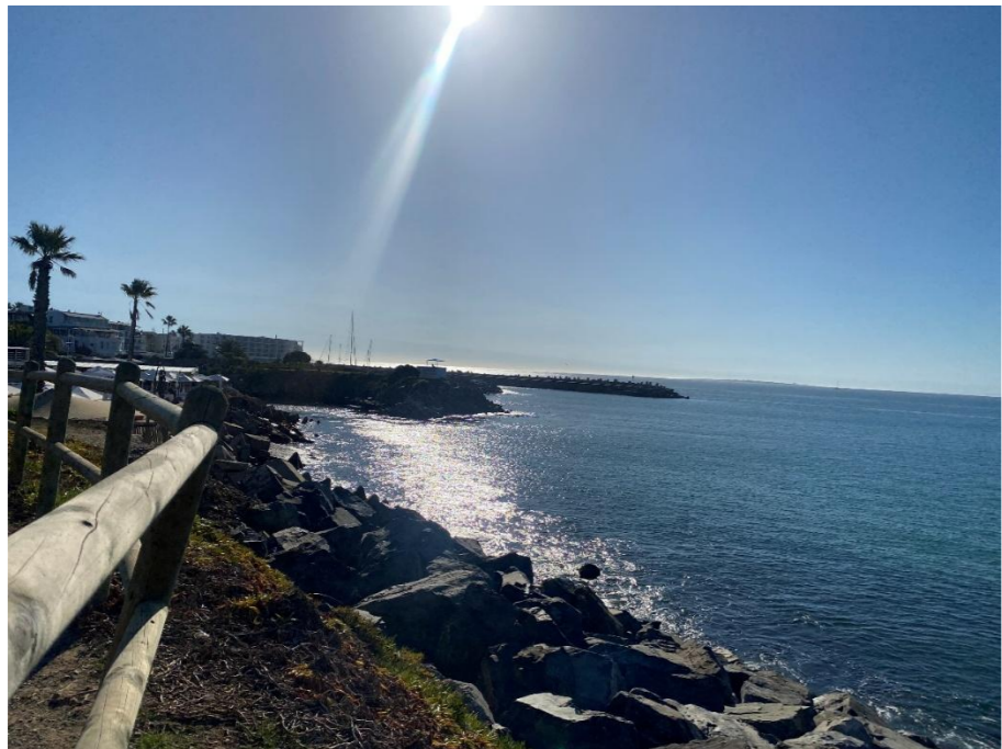
Photograph 3-10: Area to be reclaimed showing the dolos revetment (view from the east of the site)
