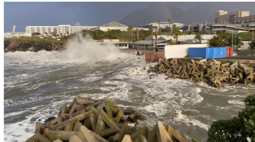
Photograph 4-5: Overtopping in front of Grand Café and Beach on 13 July 2020 (exact time unknown). Photo credit: Anton Holtzhausen (PRDW, 2023)
