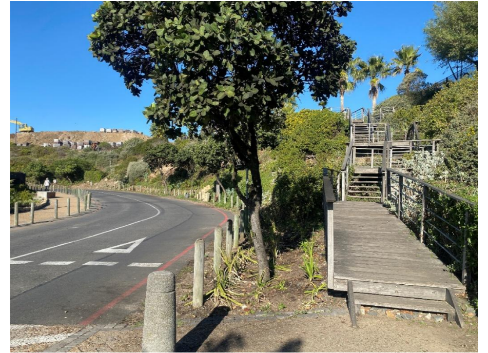
Photograph 3-9: Pedestrian walkway next to Haul Road (left) and stairway to the parking structure (right)
