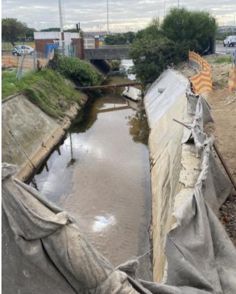
PHOTO 13: Silt screen between the works area and the Theo Marais Canal
