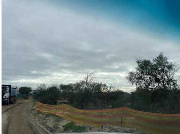
PHOTO 21: Demarcation of the sensitive indigenous vegetation adjacent to work site and access road
