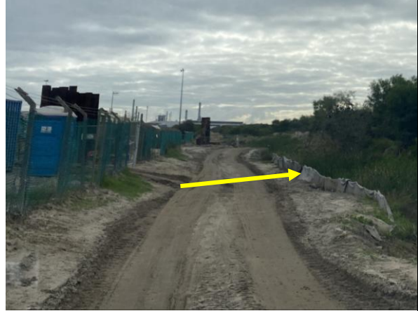
PHOTO 14: Silt screen next to stormwater channel
