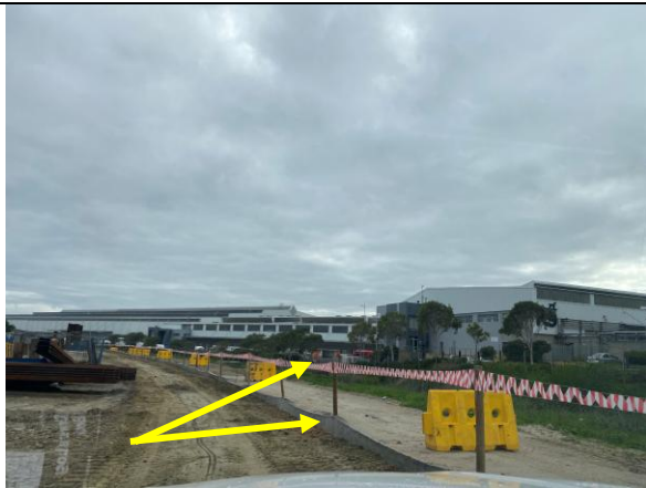
PHOTO 15: Duikersvlei buffer fencing and silt screen
