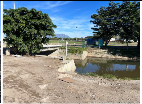
PHOTO 20: Work site cleaned next to the Theo Marais Canal
