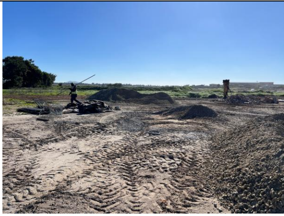
PHOTO 19: Theo Marais waste management and laydown area being cleaned up
