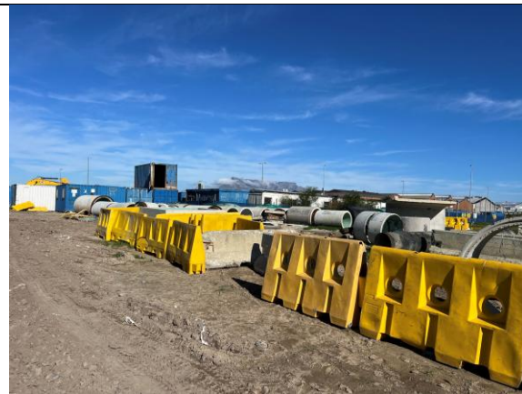
PHOTO 4: Laydown area next to site office (will either be removed or retained for next phase of work)
