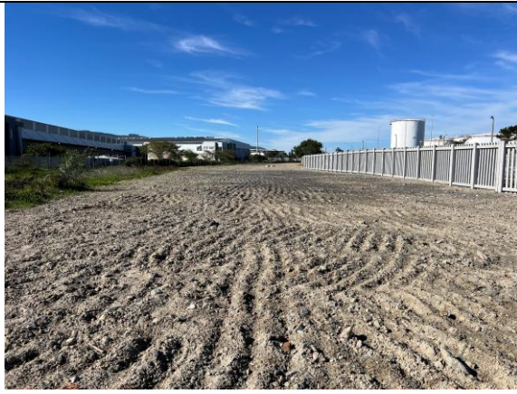
PHOTO 7: Looking towards MH 37 (wetland far left) – the area has been cleaned, graded and seeded.
