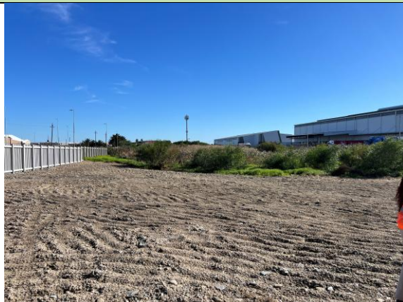
PHOTO 5: Looking towards MH 35 and wetland beyond – the area has been cleaned, graded and seeded.
