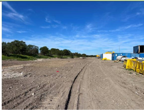
PHOTO 12: Area next to the site office laydown area cleaned up and graded
