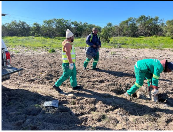
PHOTO 13: Final cleanup of the site in progress
