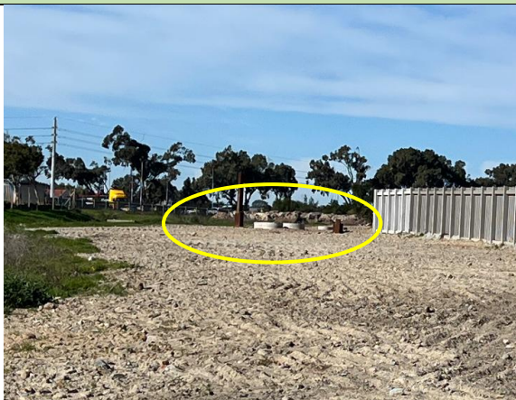
PHOTO 11: Stockpiles still to be removed
