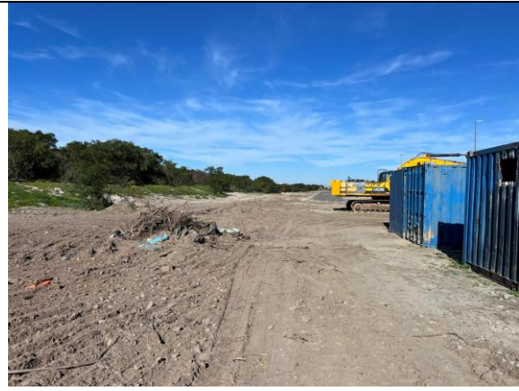
PHOTO 14: Cleanup of the area near the laydown/site office area, final waste being removed
