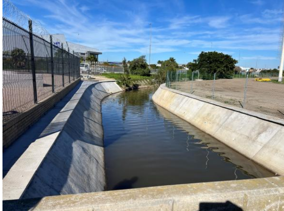
PHOTO 17: Theo Marais Canal repair completed under a separate City of Cape Town management approval.
