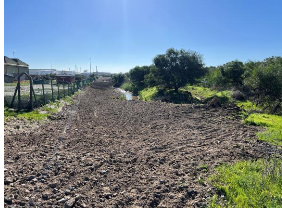
PHOTO 10: Duikersvlei canal and sensitive vegetation area to the right – undisturbed and adjacent area cleaned and ripped to allow for rain infiltration and natural revegetation
