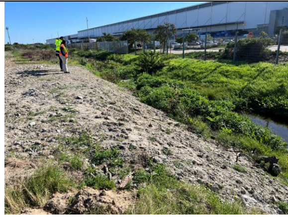
PHOTO 8: Wetland edge and repaired embankment, seeded for revegetation
