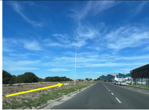
PHOTO 16: Railway Road work site cleaned and graded
