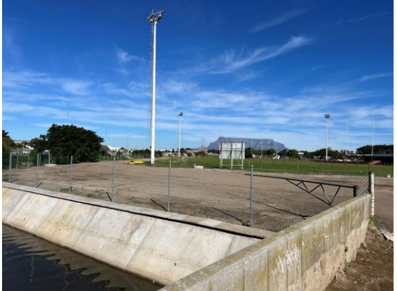
PHOTO 18: Theo Marais Sports complex work site cleaned
