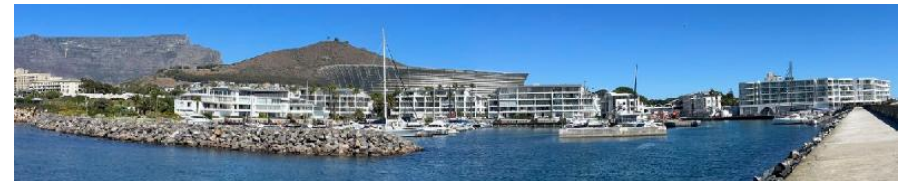
Figure 36: Neighbouring The Water Club and The Radisson Hotel to the west of the site (MALA)
