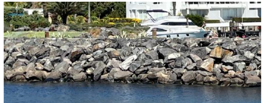
Figure 72: Preferred revetment using large rocks (MALA)
