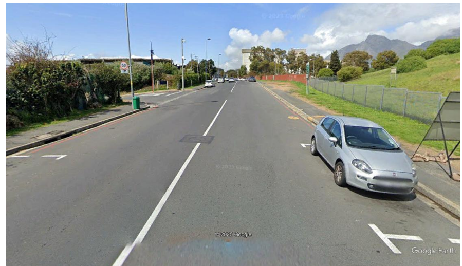
Figure 26: Beach Road east bound, access to Oceana Club and OZCF Market left, Fort Wynyard right (Google Earth).
