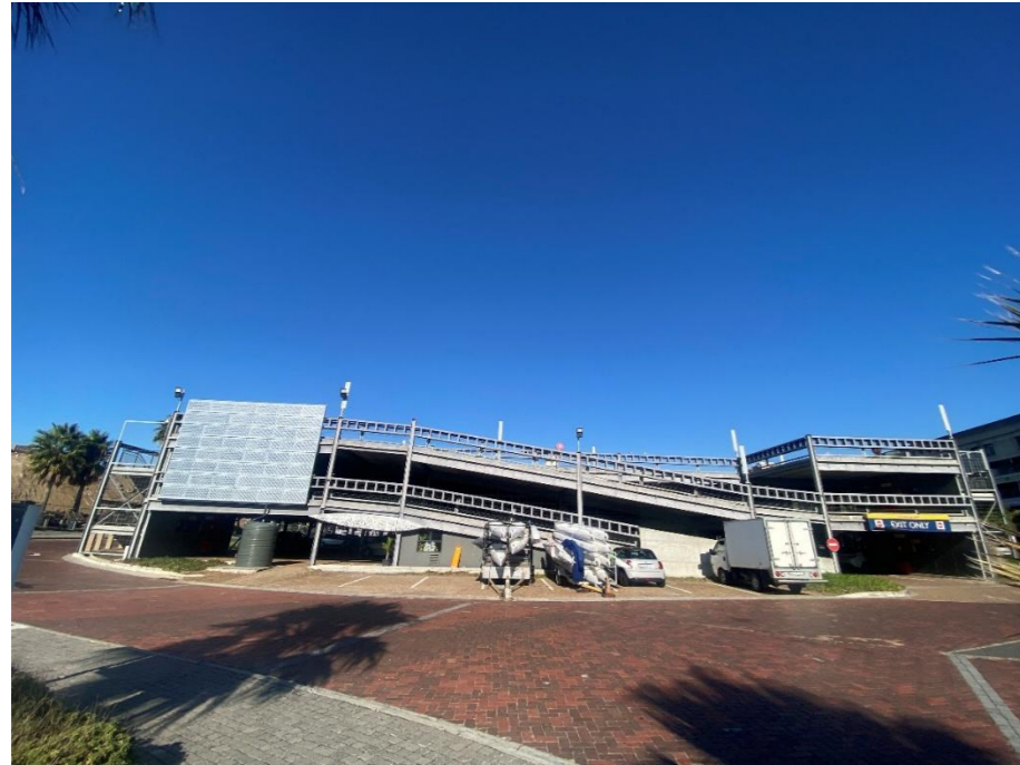
Photograph 3-7: Three-story parking structure adjacent to the former Oranjezicht City Farm Market site
