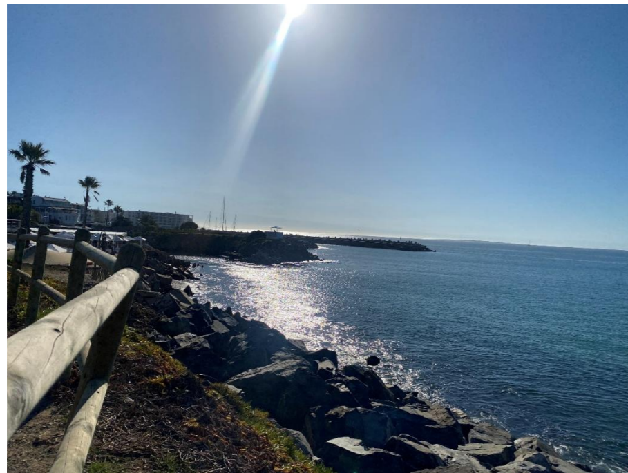
Photograph 3-10: Area to be reclaimed showing the dolos revetment (view from the east of the site)
