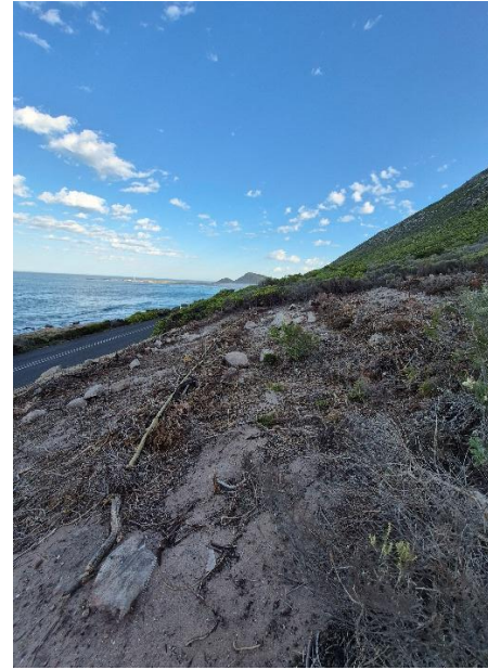
Photograph 12: Cut branches stacked in secure piles to create natural contours
