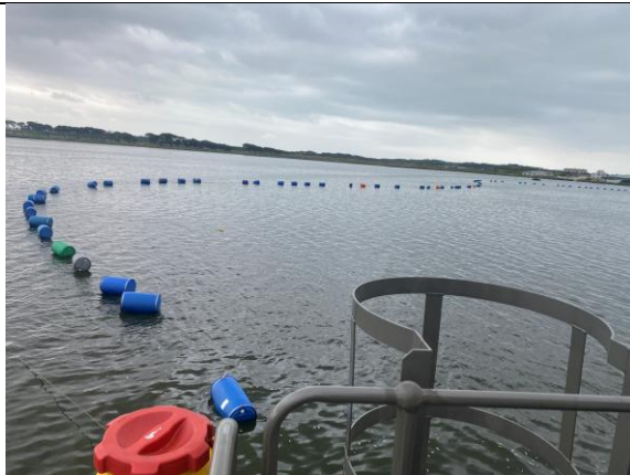
PHOTO 13: Buoys marking the pipeline in the water
