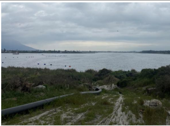
PHOTO 9 and 10: Pipe route through terrestrial vegetation area (between Billy's Block and the Zeekoevlei)– stabilised with geotextile to prevent erosion
