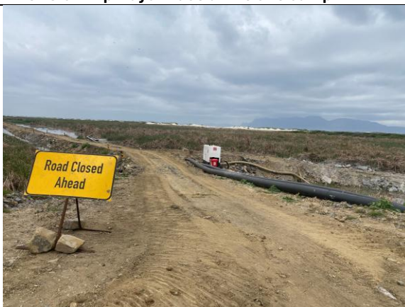
PHOTO 7: Bund wall over S3 Pond
