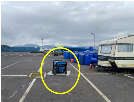
PHOTO 5: Drip trays in use at the site camp
