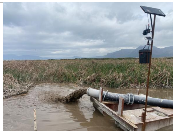
PHOTO 8: Dredging silt entering S3 pond
