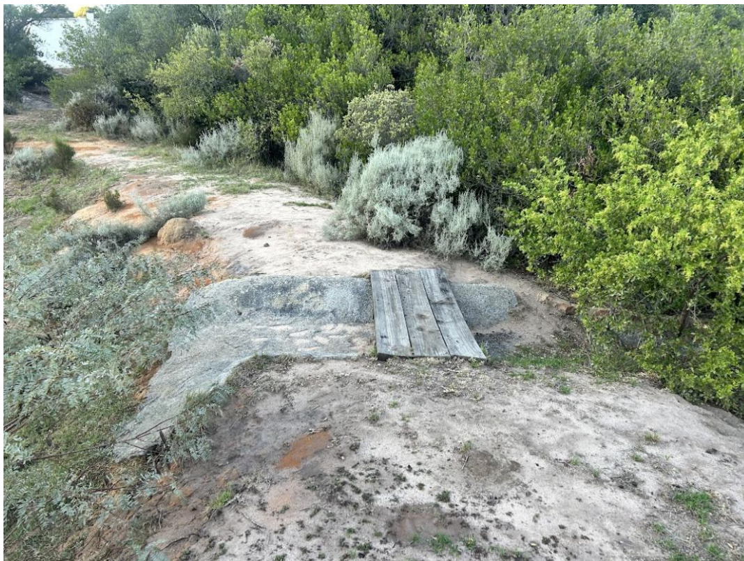
Photograph 8. Concrete spillway over the dam wall of Dam 4
