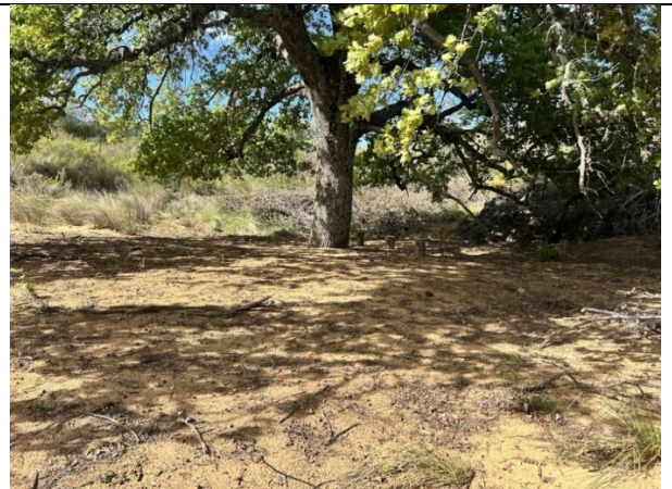
Photograph 6: Sediment accumulated within Dam 5.
