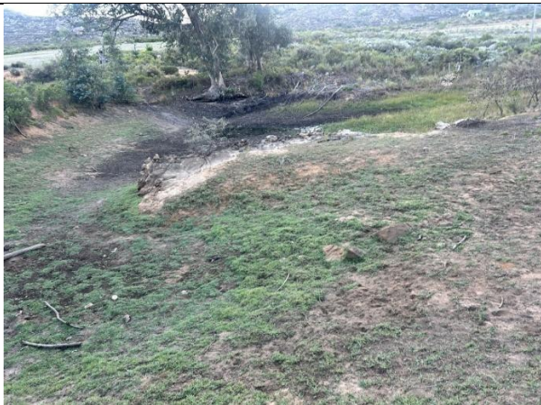
Photograph 5: Existing condition of Dam 4 (April 2026).
